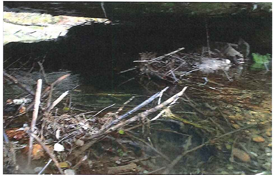
CK2262 From Downstream
